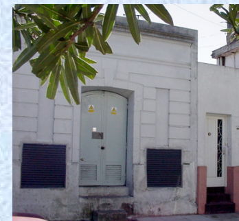
CT3: underground MV/LV
